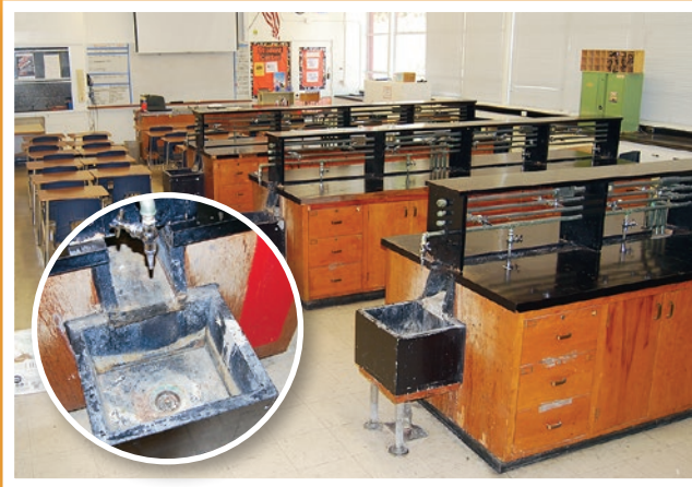
▲ Modernize science labs to improve student achievement in science and technology.
